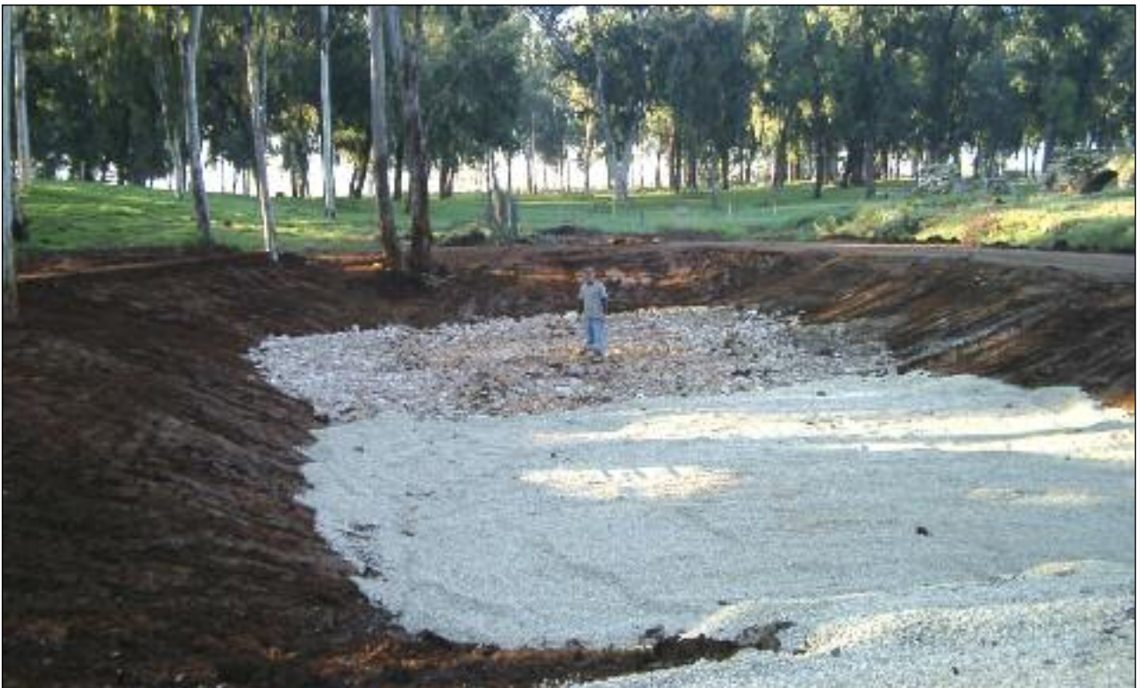
Fig. 11. The engineered bottom of the experimental side pond near Yarqon River. Picture by Y. Raz.
